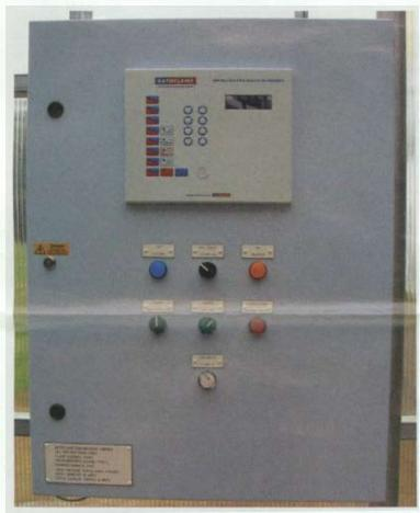
The biggest advantage of servo control is when it is coupled with a computer to control all the capabilities of a burner. For example, AutoFlame makes a control package that, when coupled with a fully modulating burner, can increase your boiler effeciencies 10-20 percent.
